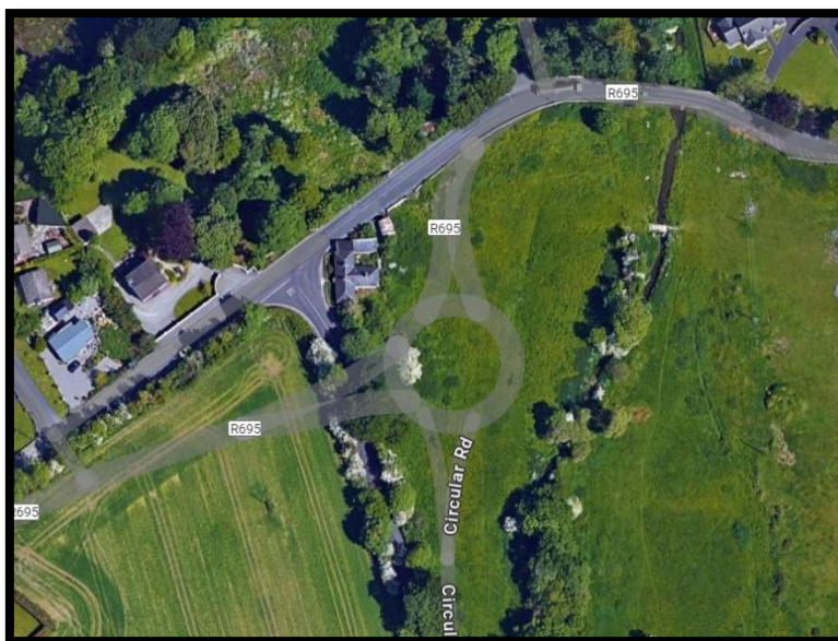
Aerial View of R695 Circular Road Roundabout @ Kilcreen
