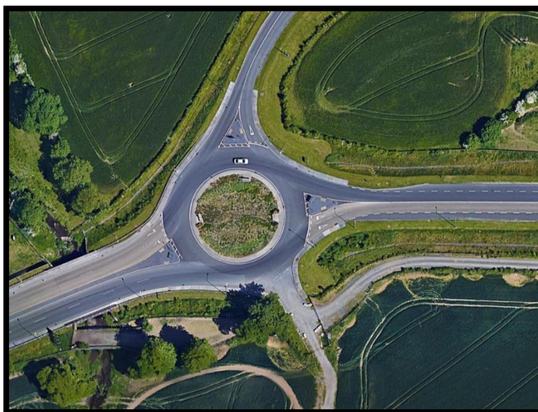
Aerial View of N77 Castlecomer Road Roundabout
