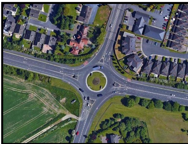
Aerial View of N10 Waterford Road Roundabout
