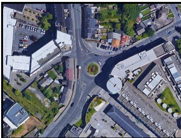
Aerial View of MacDonagh Junction Roundabout
