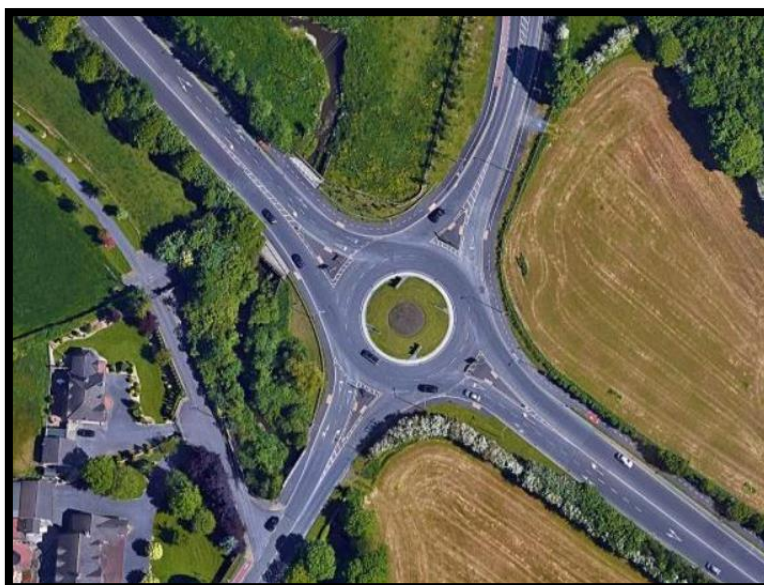
Aerial View of N76 Kells Road Roundabout
