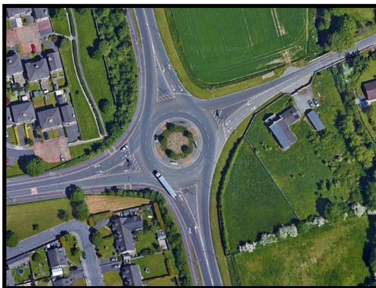
Aerial View of N77 Castlecomer Road Roundabout
