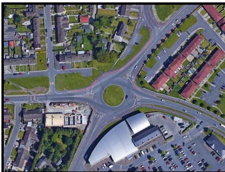
Aerial View of Newpark Drive Roundabout
