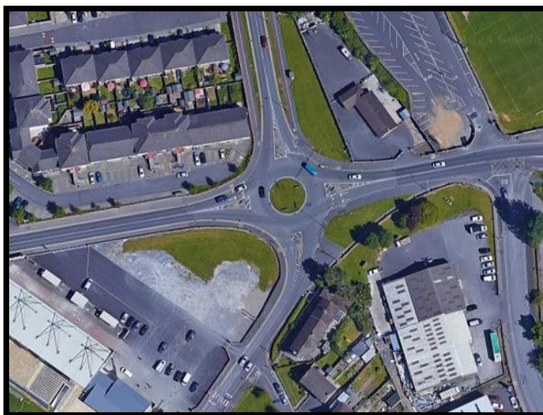
Aerial View of O’Loughlin Road Roundabout
