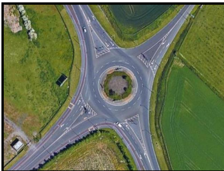
Aerial View of N77 Castlecomer Road Roundabout
