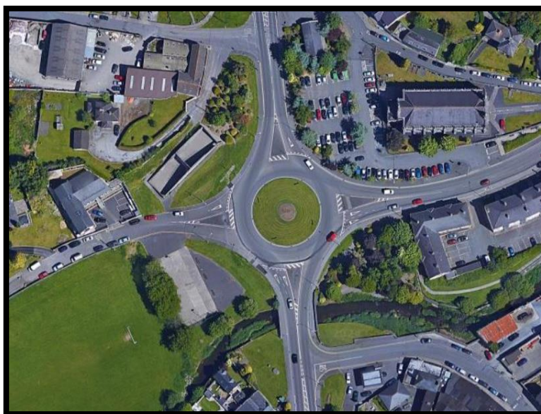
Aerial View of R695 Waterbarrack Roundabout
