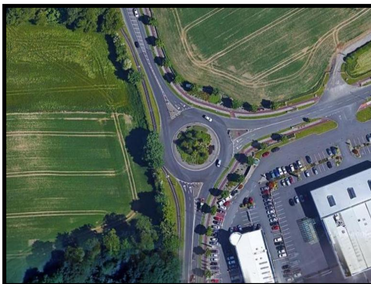
Aerial View of N10 Springhill Roundabout
