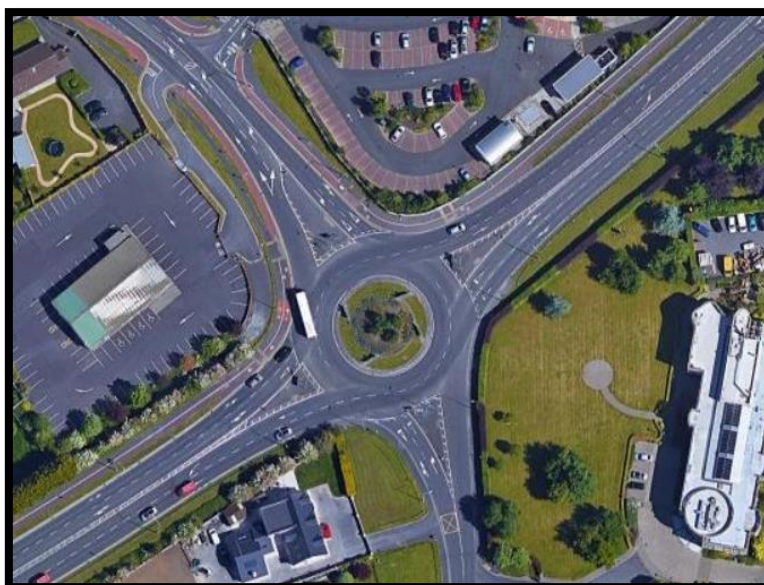
Aerial View of N10 Bohernatounish Road Roundabout
